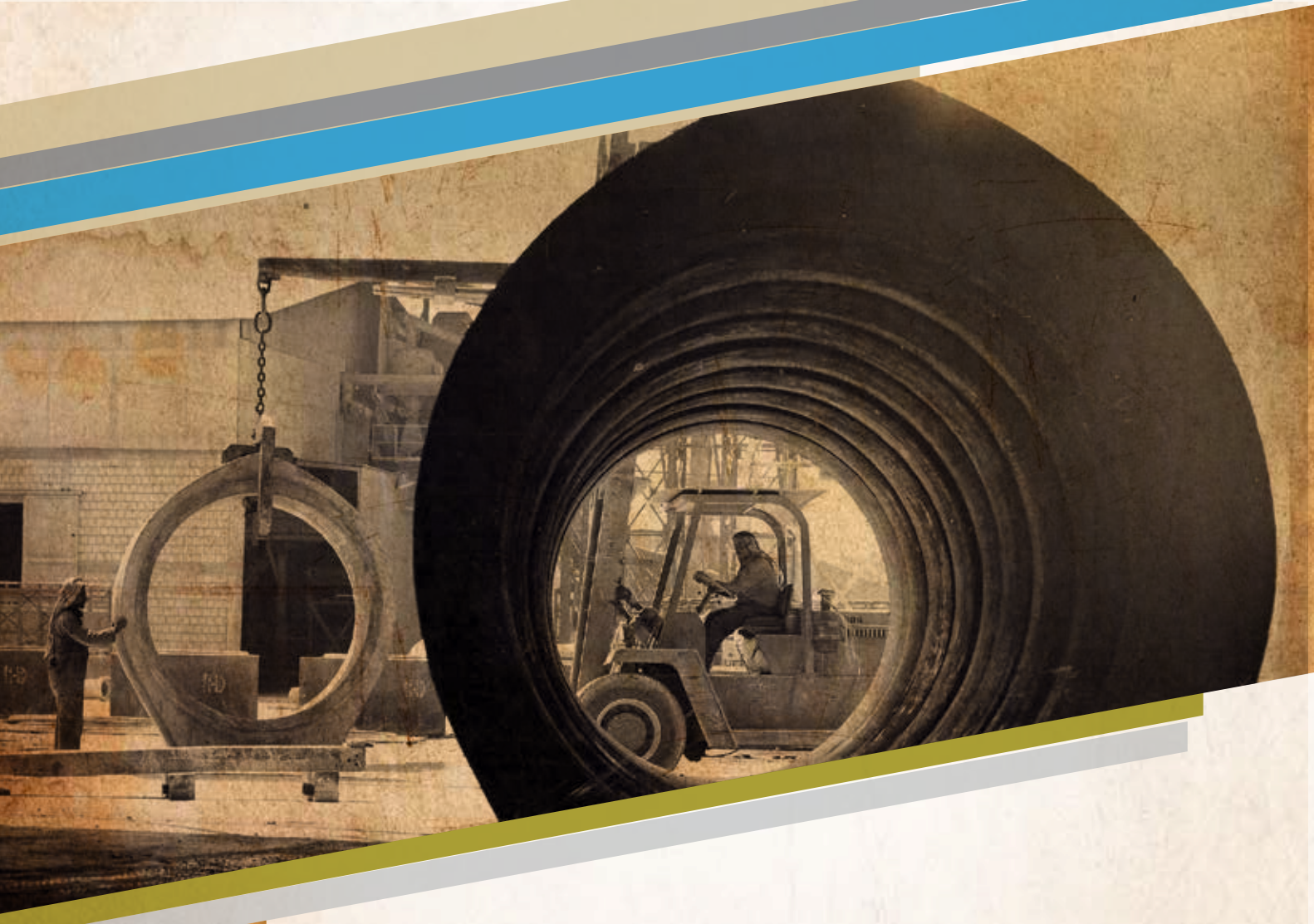
Concrete Pipes Factory after being transferred to Sulaibiya Factories Group in 80s one of the largest pipes factories in the Middle East.
